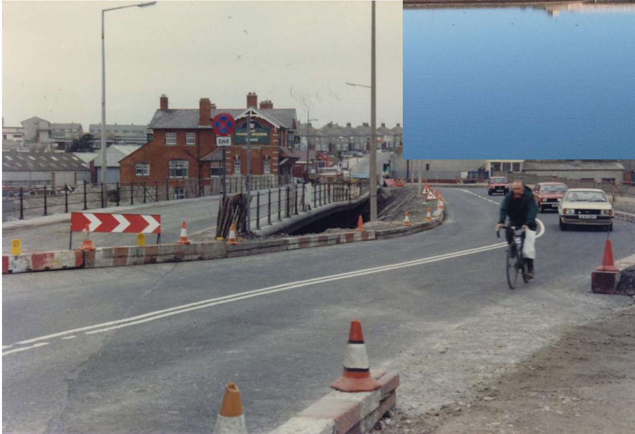
The old Victorian road bridge with the temporary road used while the new bridge was being constructed. Note the kink in the old bridge
