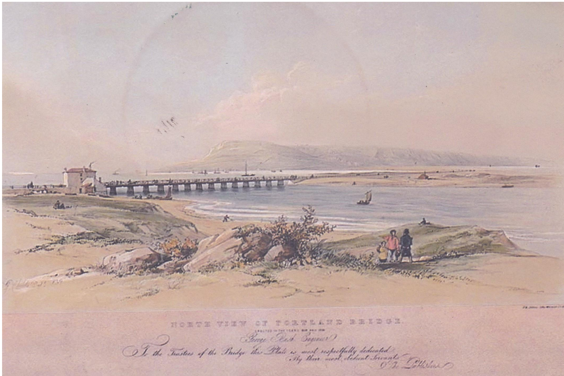
The first road bridge
